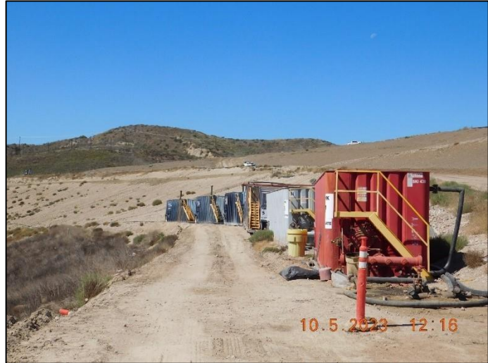
Figure 6 - Baker Tanks for temporary leachate storage.
